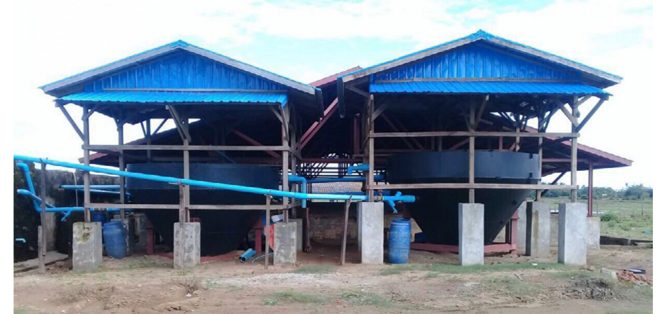
Figure 17: Hopper Bottom Tanks
