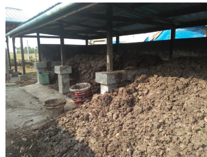
Figure 27: Dried Sludge Storage Units
