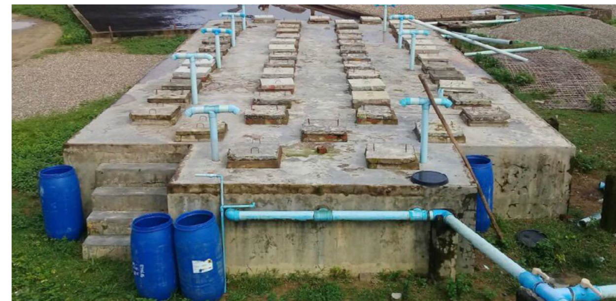
Figure 19: Anaerobic Baffled Reactor
