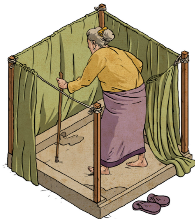
Inside the household, a concrete slab with drainage can be used as a bathing facility with the set-up of a tarpaulin for privacy, while also being useful for other purposes, such as laundry or washing dishes.
