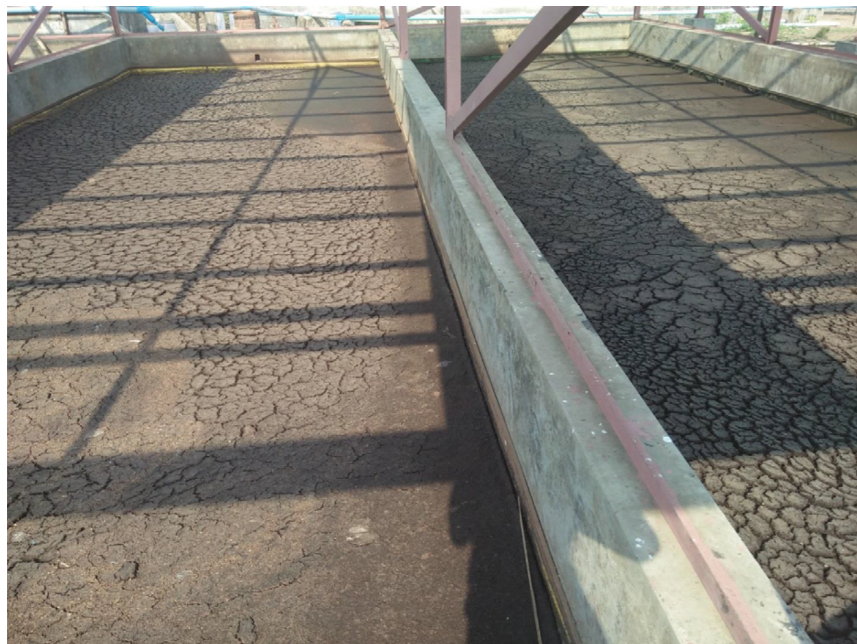
Figure 24: Unplanted Drying Beds
