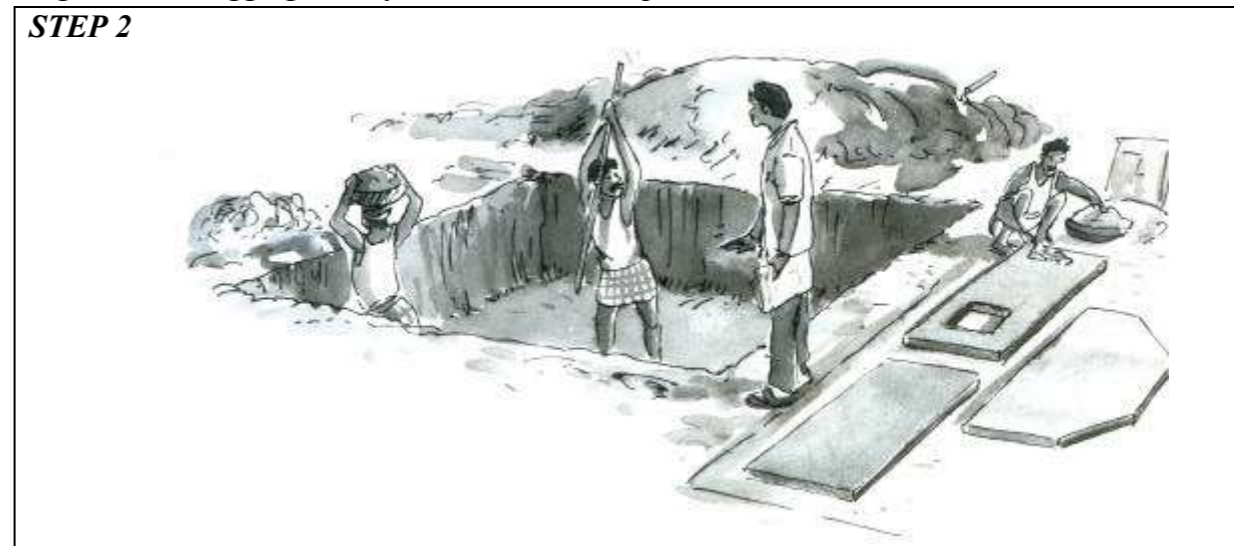
Figure 2.3.2 Digging WDU foundation and ash pit
