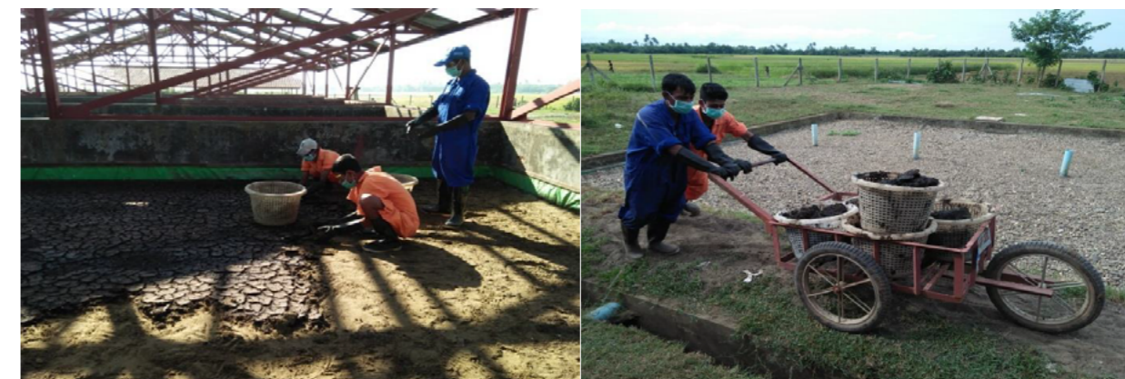
Figure 25: Workers removing and transporting dry sludge to storage
